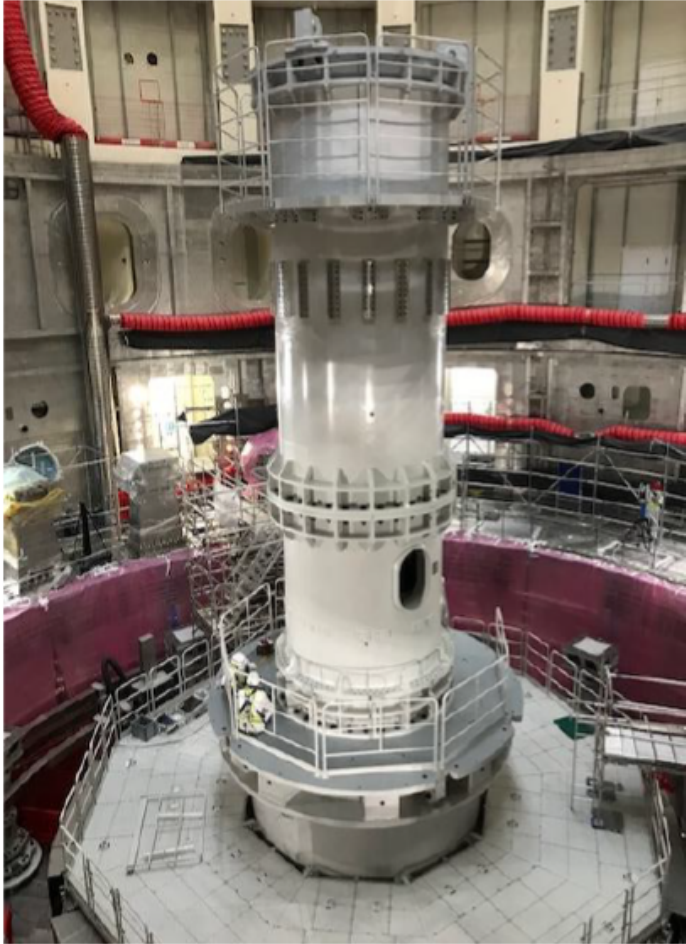
Central Column installation in the Pit
